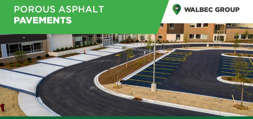
With proper mix design and routine maintenance, porous asphalt can function for decades and outlast other impervious pavement alternatives in both durability and permeability.
